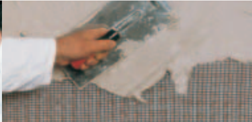
Simply lay on plaster with a trowel.
